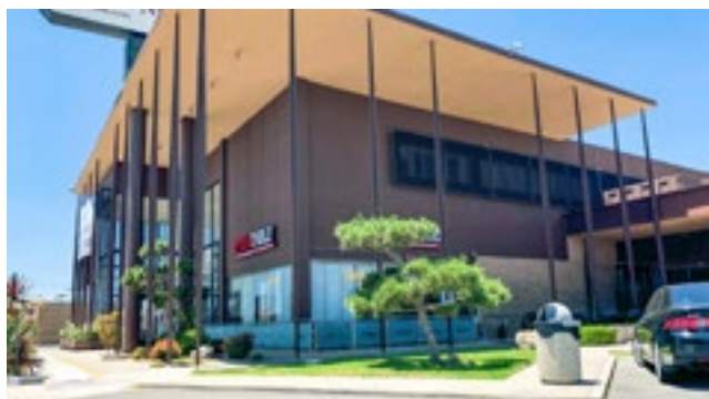
Sumitomo Bank building in Anaheim.
